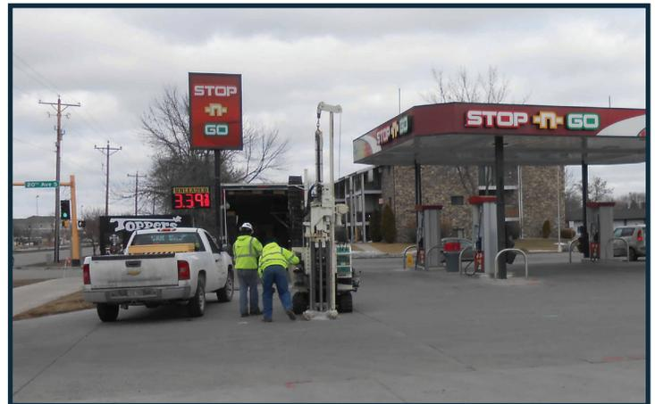
**ABOVE:** Drilling crew installs a temporary monitoring well.
