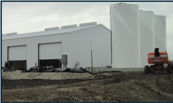
ABOVE: Bulk plant with 60' x 105' storage building.
