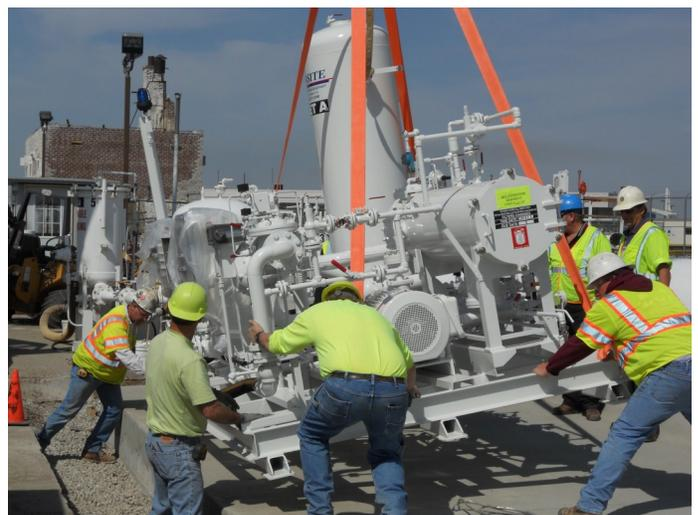
ABOVE: Installation of Phase I new Jet-A fueling skid.
