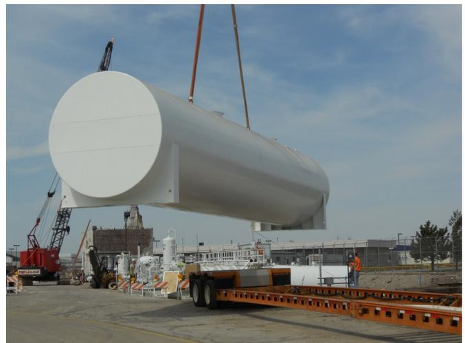
ABOVE: Delivery and setting of new 50,000 gallon Jet-A tank.
