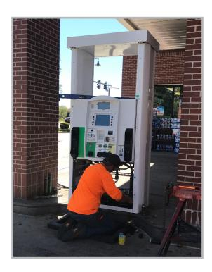
Once that is complete, an electrician re-connects power so a service technician can come through to fire up, purge and calibrate the new dispensers. A large part of Seneca's success during this project is due to expert electricians who minimize downtime by keeping up with crews disconnecting and re-connecting dispensers.
