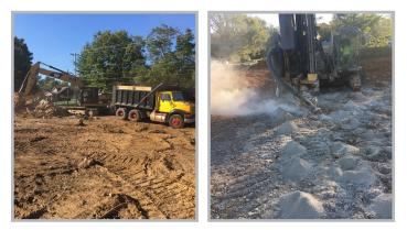
The project began with the demolition of three houses on a corner lot near US Highway 31 and Highway 100. Seneca then had to blast solid rock before digging the tank hole.
