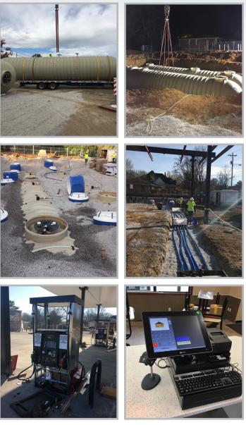
Seneca's Fuel Systems division installed the tanks, piping, dispensers and POS system. The tanks were set late at night, a result of having to blast the rock first.
