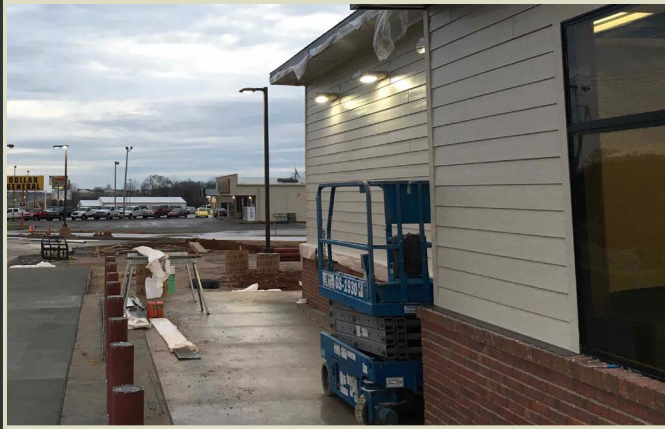
The finishing touches at a Casey's General Store in Auburn, Kentucky.
