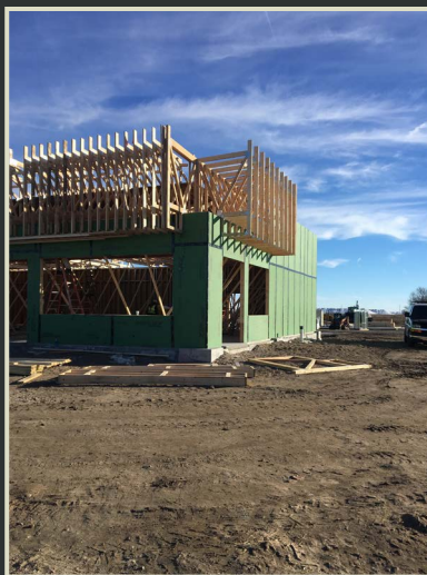
Erecting the building at Casey's General Store in Cozad, Nebraska.
