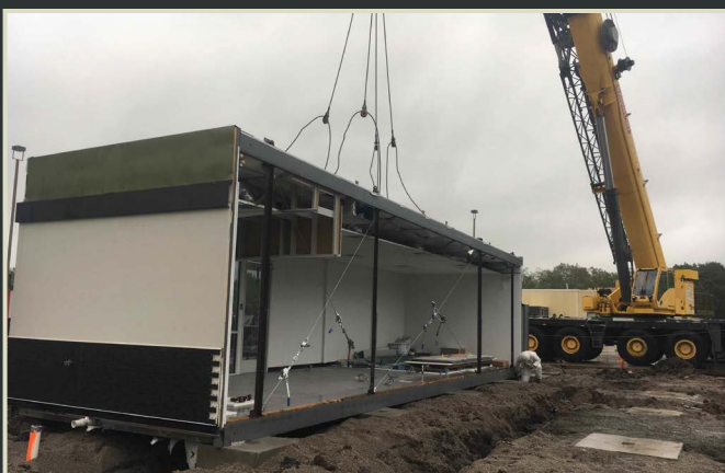
Modular c-store in progress.
