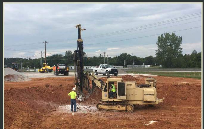
Blasting rock while constructing a Casey's General Store in Auburn, Kentucky.
