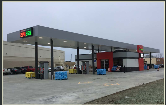
Completed modular c-store.
