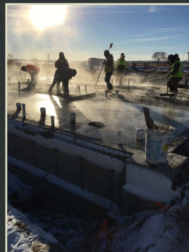
Pouring the building slab at Casey's General Store in Cozad, Nebraska.
