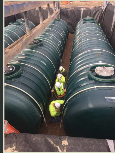
Three 30,000 gallon USTs were installed at Casey's General Store in Cozad, Nebraska.
