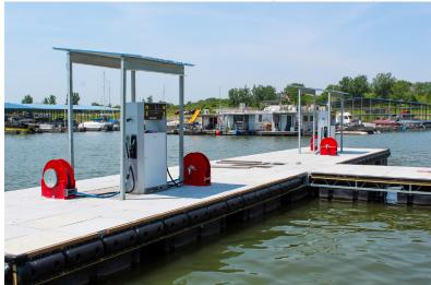
In the second phase of the project, the Seneca team completed the installation of new aboveground fuel piping from the shoreline transition sump to a newly constructed dock. This included replacing the marina's old dispensers with two new Dover Fueling Solutions<sup>®</sup> dispensers, fully integrated into the updated fuel system. The new dispensers support the marina's expanded fueling capabilities and complement the addition of the new dock and dockside restaurant.
